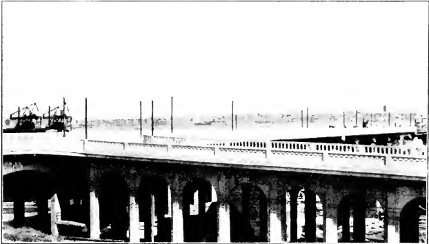
FIG. 10. SECTION 5. SECTION 4 IN BACKGROUND.
